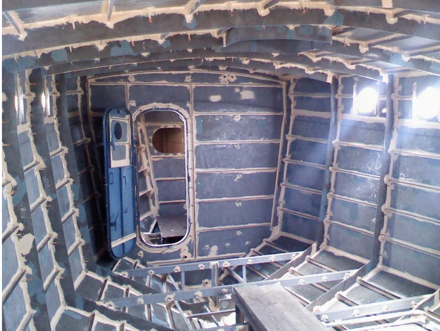
This is what proper strip coating looks like. An extra layer of paint on every edge and every joint.
